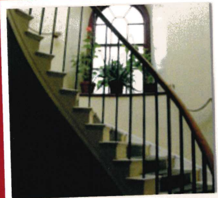
THE NEW STAIRCASE
